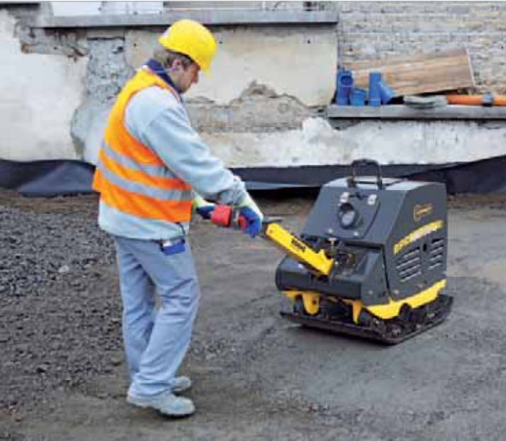
BPR 100/80 D features outstanding compaction performance on earthworks.
